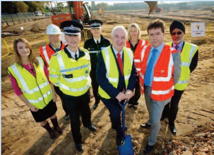
Police and Crime Commissioner David Jamieson and ACC Cann beginning construction of the new Perry Barr custody suite
